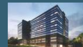
SEZ at Blue Ridge, Pune
